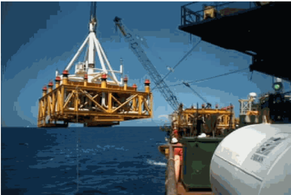
Figure B: Installation of 250 tons subsea manifold in the Marlim field .
